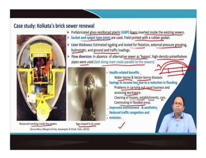
Pre-fabricated glass reinforced plastic liners were inserted inside the existing sewer. Socket and spigot type joints were used and liner thickness was estimated based on which it was tested for different kind of loads, external pressure grouting, hydrostatic tests and water leakage tests, the ground and traffic loadings tests.
