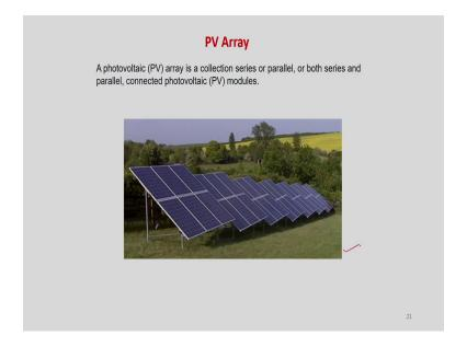
Now, if these modules, what we have discussed so far, are connected for generation of large amount of power, then it is called PV arrays. A photovoltaic array is a collection of series or parallel or both series and parallel connection or connected photovoltaic modules. So, these are the modules which are connected, and this is for a large power generation unit.
