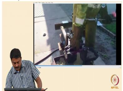
So after preheating they are coalescing the mould and then the thermit mixture is kept (Refer Slide Time: 09:29)
