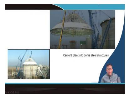
You should try to see the placement of that crown this is a area where a big failure may take place. Because this will have to be very precisely placed over the tower.
