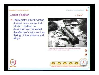
In fact, this is what the committee in UK read this and they suggested a new test to be done. And what was the new test? The Ministry of Civil Aviation decided upon a new test which in addition to decompression simulated the effects of motion such as flexing of the airframe and wings.
