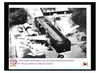
And you can see the test read.Now, it is so huge.They had constructed a water tank; the entire aircraft is submerged, and you had wings protruded out of this, and they were flexed.
