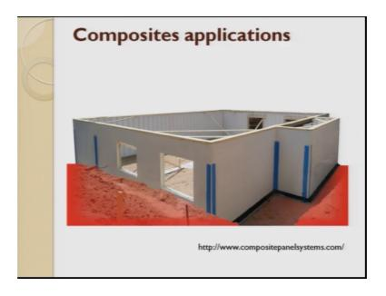
Today, houses are made out of composite materials and these houses are first it came into existence for disaster management, but today, what has happened is rapid construction are required in the third world countries. So, here, the complete roof and the side panels
