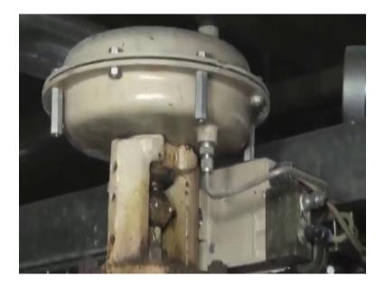
Now, this is a pneumatic valves by means of pneumatic valves, we can control the temperatures according to set point at controller.
