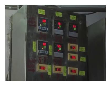
How we install the milk silo indicators and temperature indicators, where we can see the in top of the first row three level indicator indicators are installed. In first one we can see 12 where the
