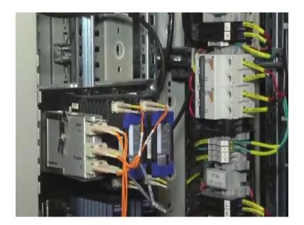
Here we can see the two control processors are there say, one question is there, why two control processors are installed heres. So, in case of one control processor fails the another one take the whole controls automatically.
