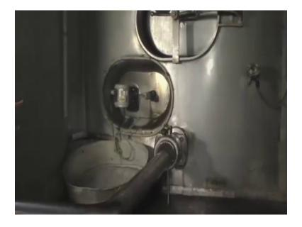
We can first see the see the what temperatures sensors called RTD sensors and this one is a hydrostatic level sensors. From wheres we take the outputs to some indicators to see the actuals level of milk in a milk silo.
