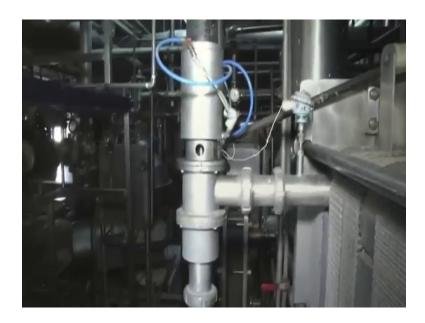
Now, here this is a diverter valve. The diverter valve is activated when the particular heating temperatures, goes below the set points ah. So, that it can be it comes into recycle area.
