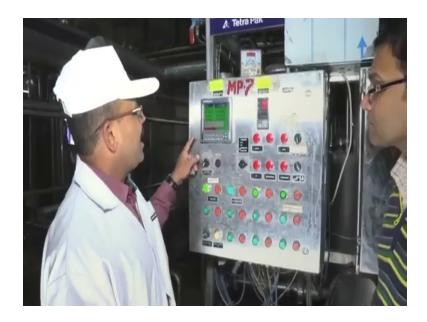
Now this is this is the temperature micro processor base level temperature controllers, and these and this is a temperature scanners.
