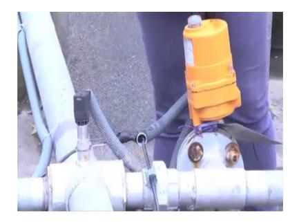
So, here for example, we have a pressure sensor installed at the junction of the pipe network to give us the pressure at this point. Likewise we have the pressure sensors at many locations of this network.
