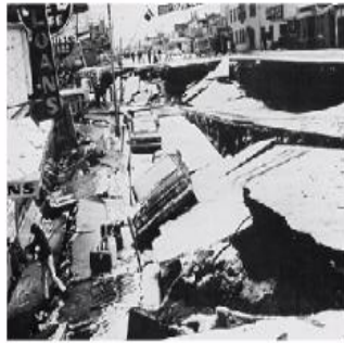
One side of this Anchorage street dropped drastically during the 1964 Good Friday earthquake.
