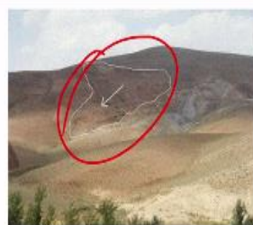
A large, ancient landslide north of the village of Estaladje
