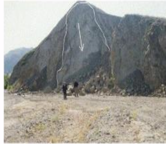
Saeed Abad rock block slide which occurred near the village of Saeed Abad. Prominent scarp on the behind of ridge crest (cannot be seen in the figure) showed as much as 10 cm downslope displacement. The pile of boulders downslope from the outlined area is due to a rock slide and several rock falls, which originated during the earthquake from the same slope and the right slopes.
