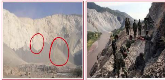
Slope failure observed in the regions of Balakot and Muzaffarabad (Pakistan Earthquake 8th Oct. 2005).
