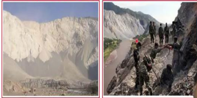
Slope failure observed in the regions of Balakot and Muzaffarabad (Pakistan Earthquake 8th Oct. 2005).
