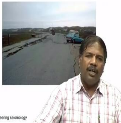
Ground failure due to liquefaction, Loma Prieta earthquake. (Photo from: http://earthquake.usgs.gov/bytopic/photos.html )
