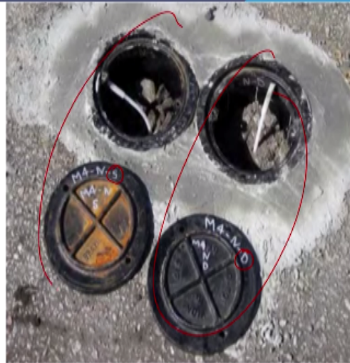
Construction of flush-mounted paired micro-wells (i.e., shallow and deep)
