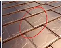
Details of the copper lining on the roof
