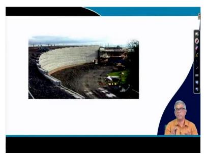
And this is the as I was telling that MSE retaining wall, this is the wall, these are actually the all facing elements and this with these facing element there are some reinforcements will be extended inside the soil and because of this weight when this wall will try to move this direction the other enforcement will have the tension in other direction. This way this entire thing will be in stable condition that analysis part we will discuss later on.
