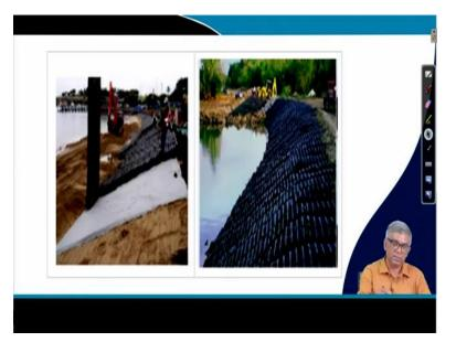
This is actually as a slope protection actually, you can see, these are the things if you put then the soil it will not direct, the water is not directly coming into because of the flow of water it eroded and this is the installation process shown in this photograph.
