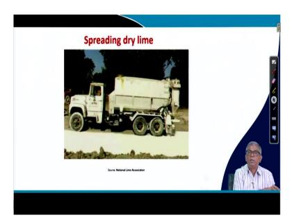
And then you have to spread the lime, of course after scarification if there is two big lamb formation is there, then you have to pulverize it. Otherwise, the big lump surface soil will react with lime but inside it will not react.
