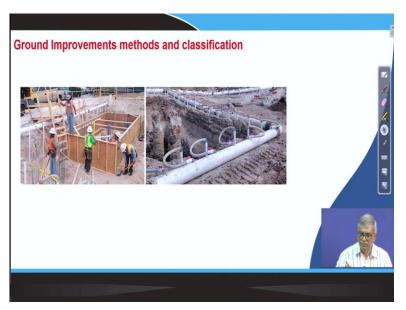
And these are the actually typical you can see here these are all well point actually these are well point this is actually different well point actually they are at well pump it is pump of different points and then through these actually water is discharged away from the construction site. So, that water table will be lowered permanently.
