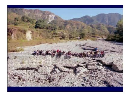
After few years this what happened ok. So, this is an another example which we can say that this is because of the seepage, which broke the wall underneath the top wall remain as it is. So, this is an another example of the landslip or the erosion which take place within the river valley.
