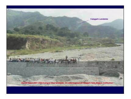
So, this is a retaining wall and as I was talking about the road which was been constructed connecting the banks on either side, again the same in the similar way this retaining wall was been put on the riverbed without having proper foundation. So, to allow the water which has been seeped within the sediments here, there are some outlets which have been put here, but that way those were not enough.
