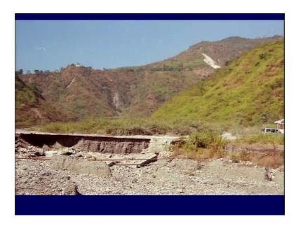
Very good example another one from Himalayas. Now if you see here what this is an riverbed here and the road which has been constructed is on the top of the riverbed just. They have filled up this much a ocean here and constructed a concrete road. Now there is an undercutting or erosion which will keep on taking place because they if you are not having the overflow from the top, but the water will keep on seeping from below. Again
