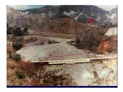
So, another good example from Dehradun region, what we see here is the channel which is flowing in this region and a bridge over here the problems which have been faced is that every time there is an excess amount of sediment bed load coming during the floods and covering this the bridge. It can damage this because this is the only connecting bridge, at that point of time this photograph was probably taken during 1970s which used to go to Missouri.
