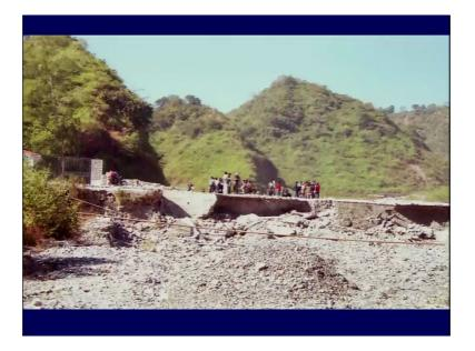
And most of the time what we find is that such roads, which are been constructed connecting the either banks will be eroded a very quickly. So, they may last for couple of seasons and then again you will have to do the reconstruction of such roads or transportation.
