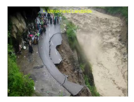
Landslides in Uttarakhand again because of the undercutting of the riverbank.
