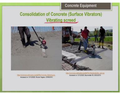
So, another type of surface vibrator is screed type vibrator vibrating screed. Screed in the sense it is a kind of finishing operation. Screeding refers to the finishing operation. In this vibrator, what we do is we do the finishing as well as the consolidation together. So, you can see the picture. So, it is doing the screeding job as well as the consolidation together. That means screeding is nothing but just removes excess layer of concrete on the top surface of the concrete and level it.
