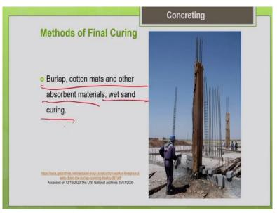
So, this picture again shows the curing based on application of water you can see they are covering with wet gunny bags, wet burlap or cotton mats, any absorbent material you can put particularly for the vertical elements. We can like columns we can go for this kind of method. So, for the slabs, we can follow ponding or immersion method. We can allow the water to stagnate easily.
