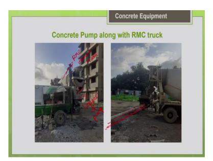
So, this picture shows you the concrete pump along with the RMC transit mixer. So, you can see this is the RMC transit mixer. This is your RMC transit mixer. So, it is delivering the concrete through the chute. The transit mixer will have a chute. With the help of the chute it is delivering the concrete into the hopper of the pump. So, from the pump, as we discussed based upon the piston action, the concrete will be delivered into the delivery pipelines.
