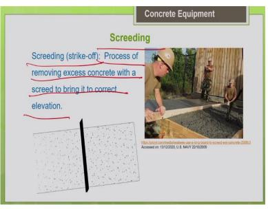
Now, let us see, what are all the different stages of the finishing of the concrete? The first step is screeding. Screeding is nothing but strike off. You can see the picture what they are doing. So, with the wooden screed, they are just trying to remove the excess concrete from the surface and level it to the right elevation or level it to a correct level. That is what they are trying to do here, so, the process of removing the excess concrete with a screed to bring it to a correct elevation.
