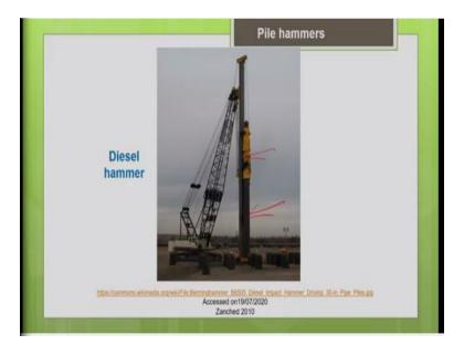
Let us see the picture of this diesel hammer you can see, this is a picture of the diesel hammer lifted by a crane. So, it is driving a steel pile, you can see this is a diesel hammer, this is a pile, it is lifted with the help of your crane.
