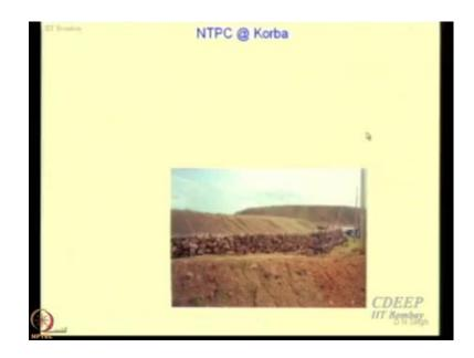
From a near distance looks like this; so, these are the mounds of the over burden. Over burden is nothing but the top soil which has to be removed before you dig the coal from the mines and it may range from 2 meters to 3 meters to 4 meters depending upon your luck and depending upon the circumstances. So, in order to get certain amount of coal you have to remove that top soil and that volume could be of this magnitude.
