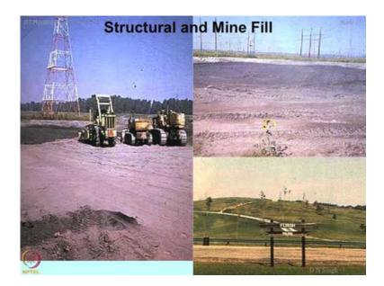
You can use this material for structural and mine fills. So, these are the open cast mines which are being filled with the help of the fly ash.
