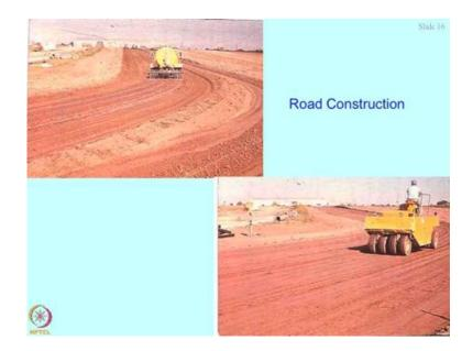
These are the examples from road construction, I am sure you must have heard of road construction using fly ash either by direct disposal on the ground compacting it putting some water and doing some pneumatic rolling all right these are all old techniques.
