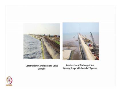
So, this is the geotextile tube which is let down near to the seashore or artificial lake. You can you can construct the artificial lake when there is no space and you want to make use
