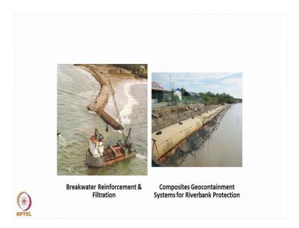
You can use for the Breakwater Reinforcement and the Filtration. You can use Composite or the Geocontainment System in the Riverbank Protection. You can see many soil is eroded many places around the wall, you can use for the geocomposite material or geo container system for the riverbank protection. This is another, their construction for artificial island using geotextile tube.
