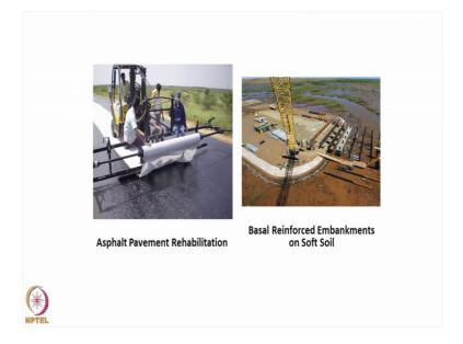
You can use here the geosynthetic material for the Asphalt Pavement Rehabilitation. You find in Bombay, many places also surrounding many places across the world and in India you can fly there is a lot of reflection cracking and the photol; you can make use of this geosynthetic material to prevent the cracking. So, here is shown an Asphalt Pavement Rehabilitation and how it can be used for geosynthetics material.
