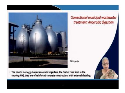
These are examples of egg-shaped digesters in the UK. This is from the Internet, from Wikipedia. So, you can see that the cladding; this is provided with cladding, and that is simply to provide insulation and keep the heat within the digester. Remember, a lot of heat is being generated in the anaerobic digestion process and it is useful heat. So, that heat has to be kept trapped within the digester, to help the efficiency and to improve the efficiency of the digestion process. So, that is it.
